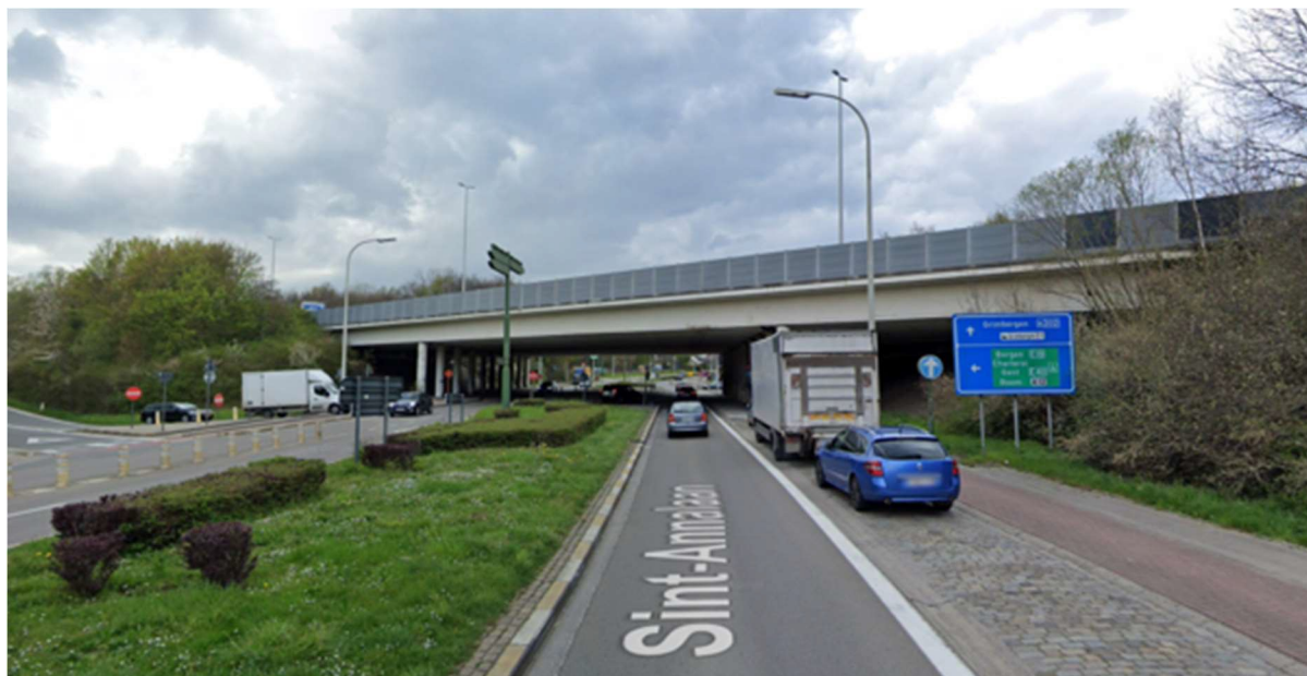
Figure 288 : Image de l'Avenue Sainte-Anne - situation existante (source : Google Maps)
